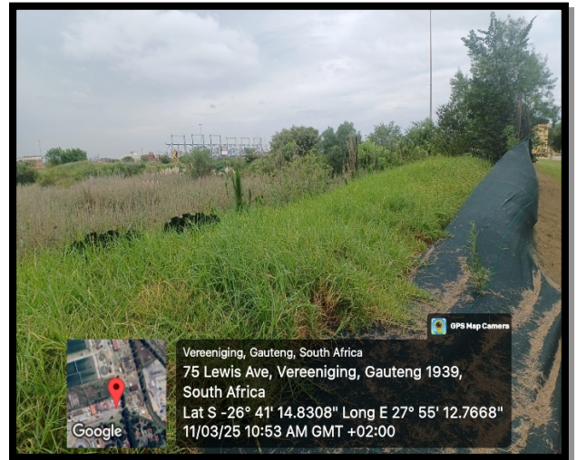
Figure 2: The Demolished Old New System 1 site
